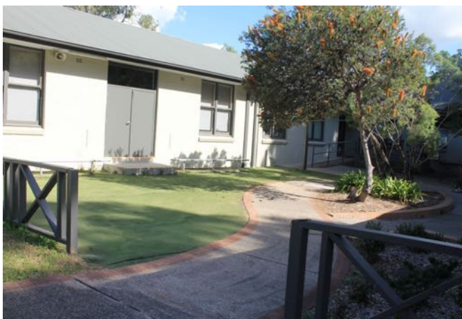
Block A, viewed to the south-west with the landscaping between it and Block D
