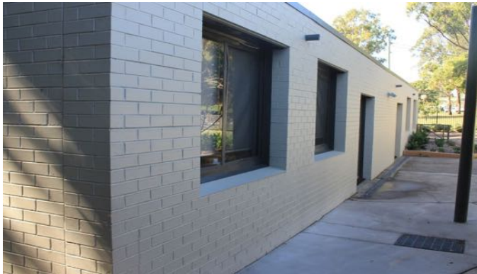
View of the southern side of Block D looking east
